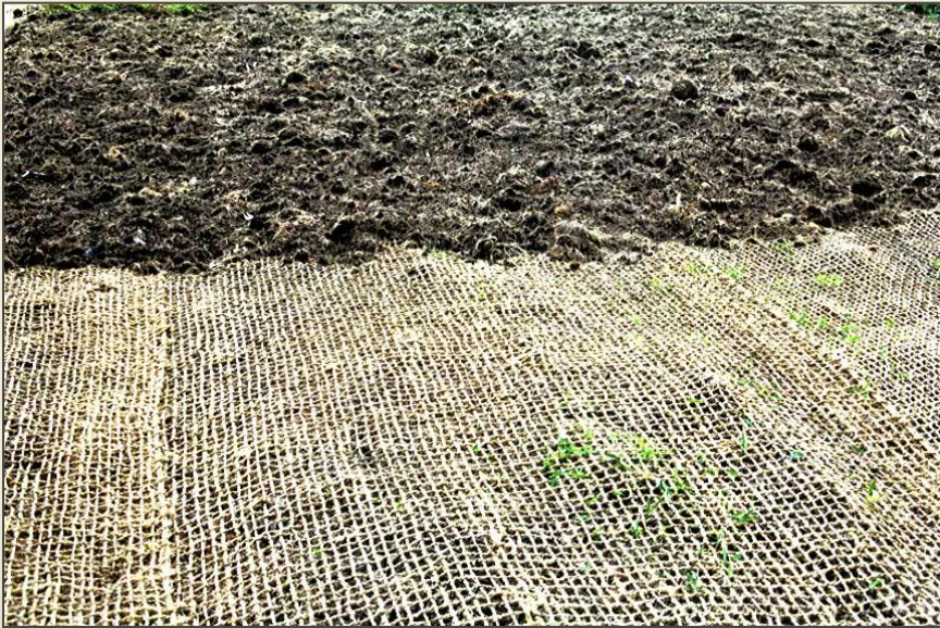
Installation of CGT over rocky patches
