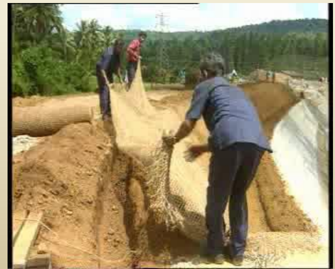
Laying of geotextiles
