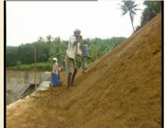
Laying of geotextiles
